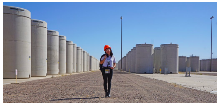
Dry cask storage at the Palo Verde nuclear plant in Arizona
